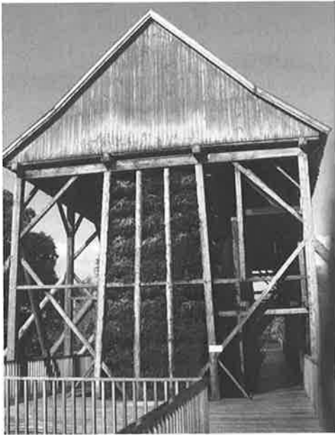
The restored section of a thornbush tower at Bentlage, Germany.
