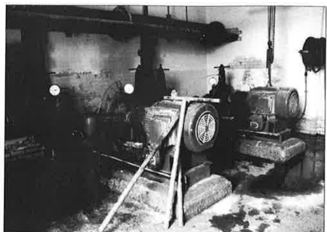
Pumps send raw brine to Middlewich.
